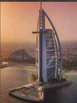
Burj al-Arab Abu Dhabi United Arab Emirates
